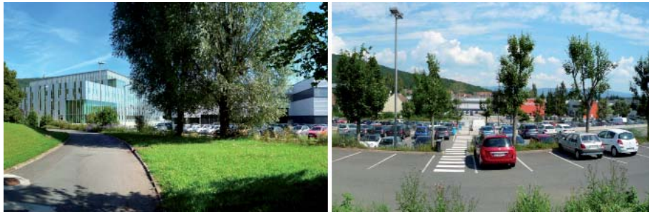
Zone UYb, site Techn'Hom 5
